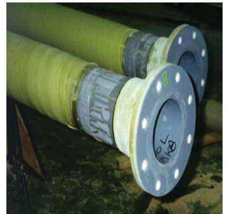
Fiberglass reinforced PVC flanged spool piece.
