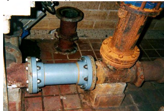
Figure 3 Uncorroded plastic pipe
