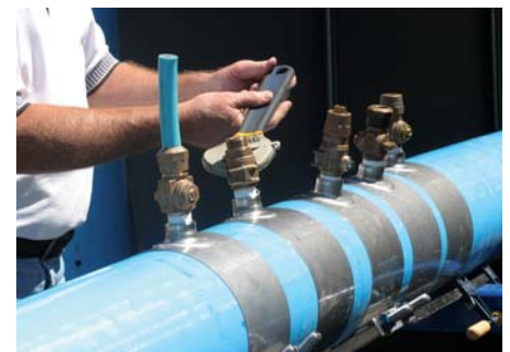
Tapping PVCO pipe is quicker and stronger than PVC pipe.
