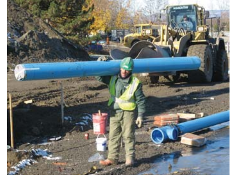
Man carrying a 20-foot length of 10-inch PVCO pipe.
