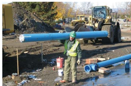
Installer carrying a 20-foot length of 10-inch PVC water main piping.
